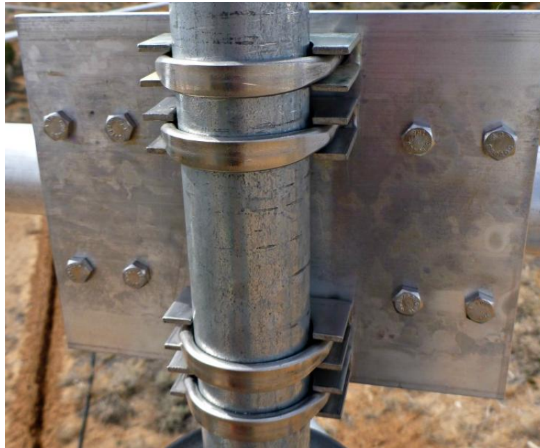
Picture of Mast Plate to Mast (Custom made Tight Fit Stainless-Steel Flat U-Bolts)
