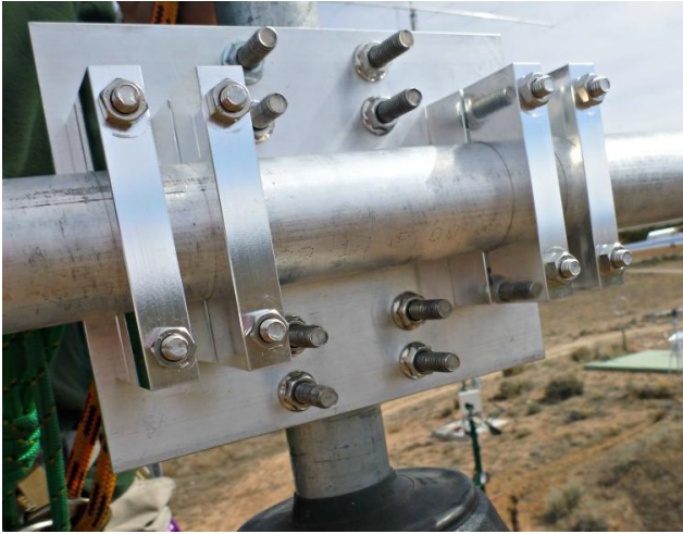
Boom to Mast Plate attached to Boom
